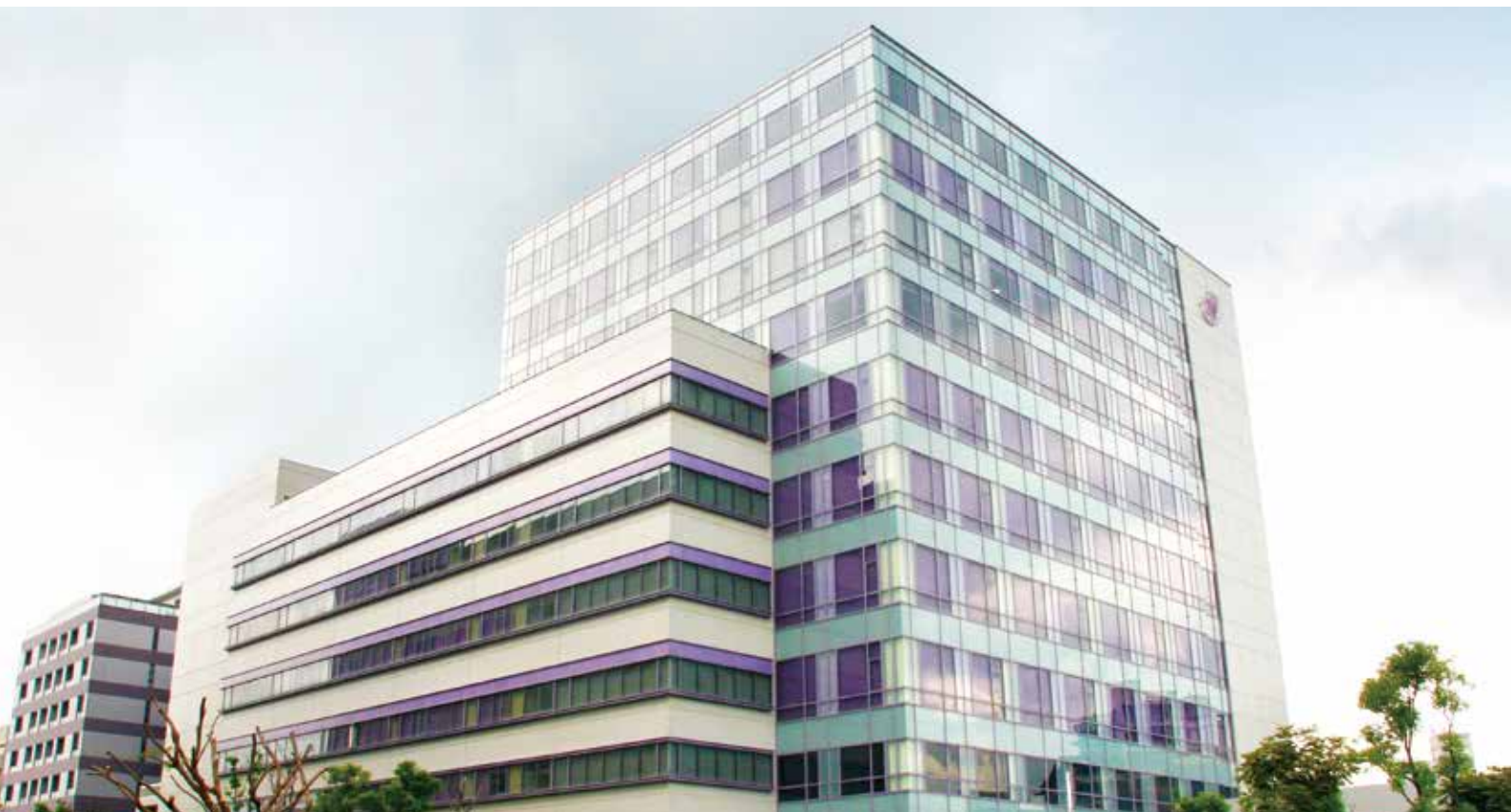
Portwell Engine (PE) Building
